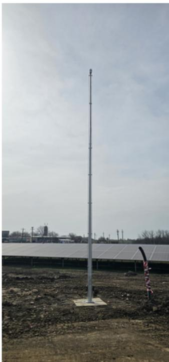
**TRV KIT COMPLET PARATRASNET PENTRU PARCURI FOTOVOLTAICE – VARF PDA 10MS, STALP 6M, 8 ELECTROZI SI CONDUCTOR OTEL ZINCAT 10 MM - ACOPERIRE CIRCULARA DE 120 METRI**
